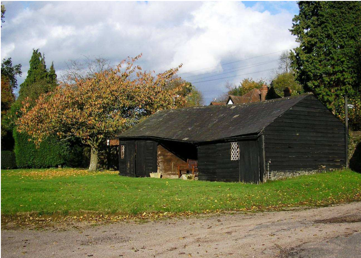
Black tarred boarding and slate roof forming a simple vernacular building
